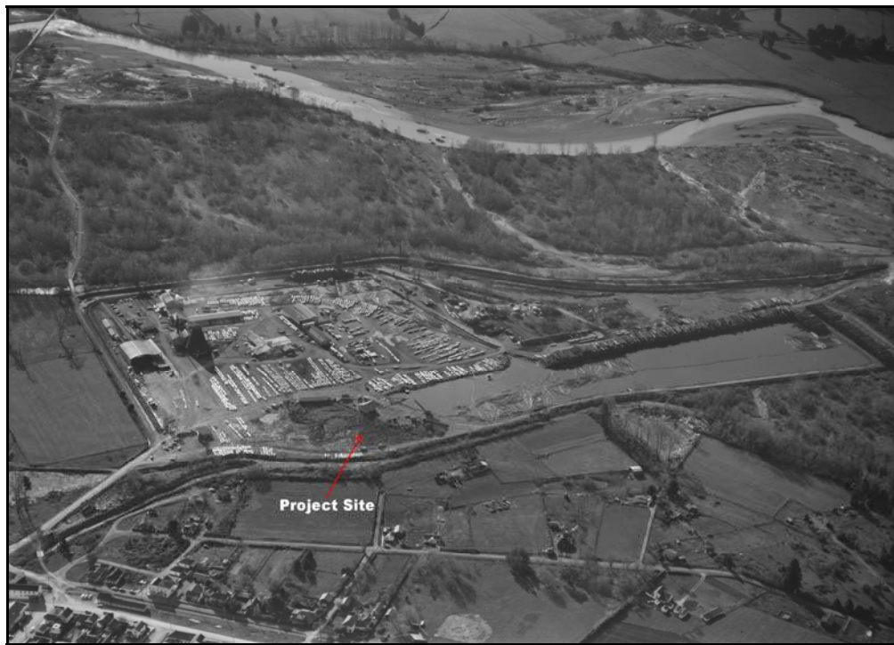
Historic Aerial Photo of the McIntosh Mill (Schuster, 1950)
