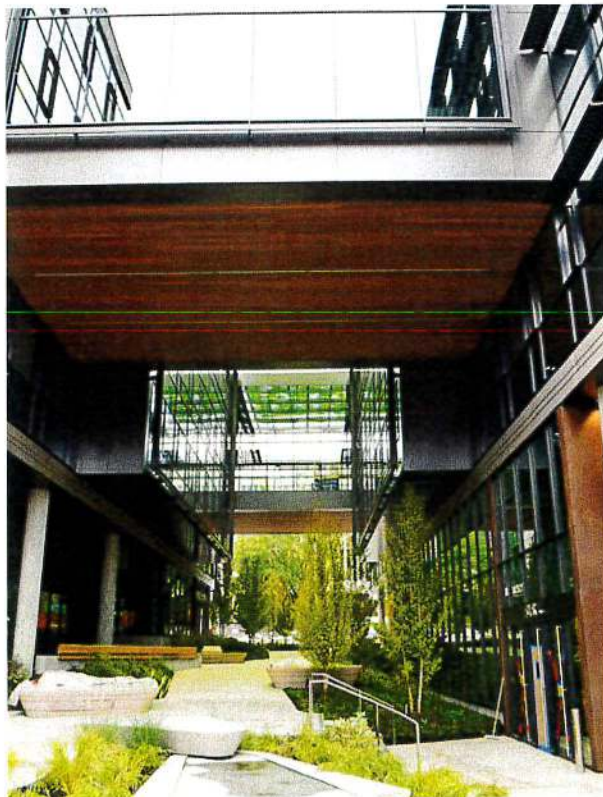
Two-story pedestrian pass-through to promote physical and visual connections, and to reduce apparent building bulk at grade level
