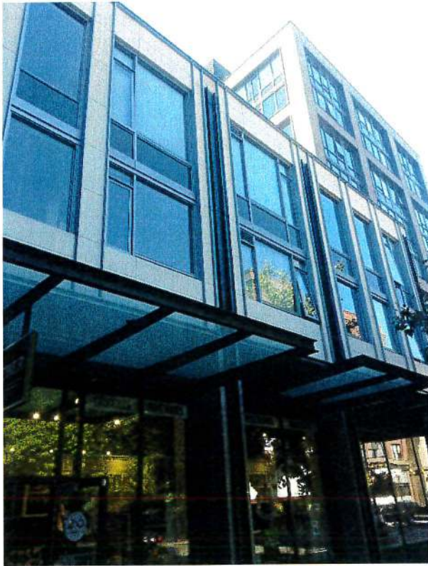
Upper levels set back from base at western edge of office building; ample glazing and canopies enhance pedestrian experience
