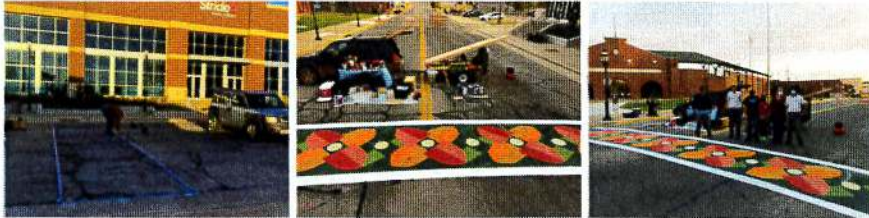
WORKING ON THE CROSSWALK
