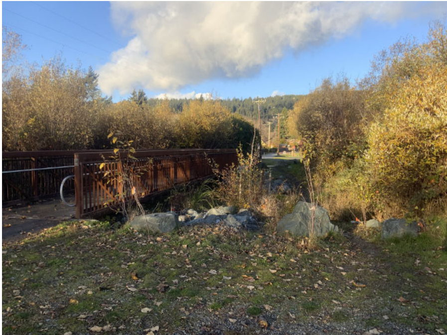
View looking north of footbridge over Powers Creek
