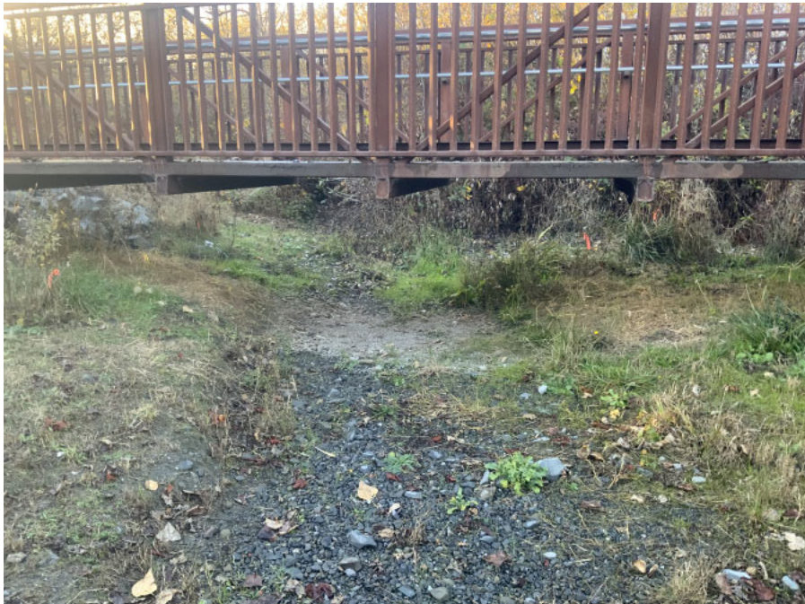
View of footbridge over Powers Creek.
