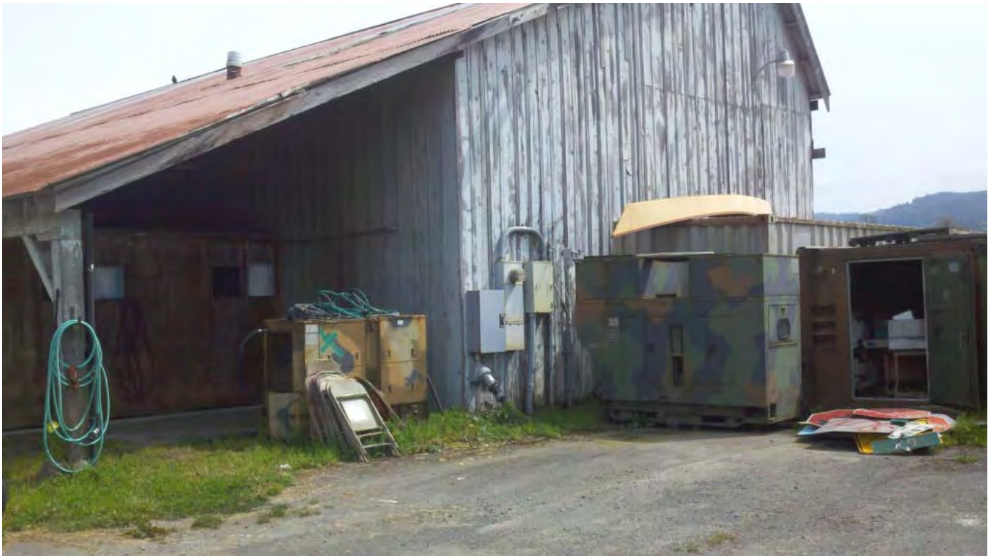
Photograph No. 26: Photo showing the northwestern side of the shop.
