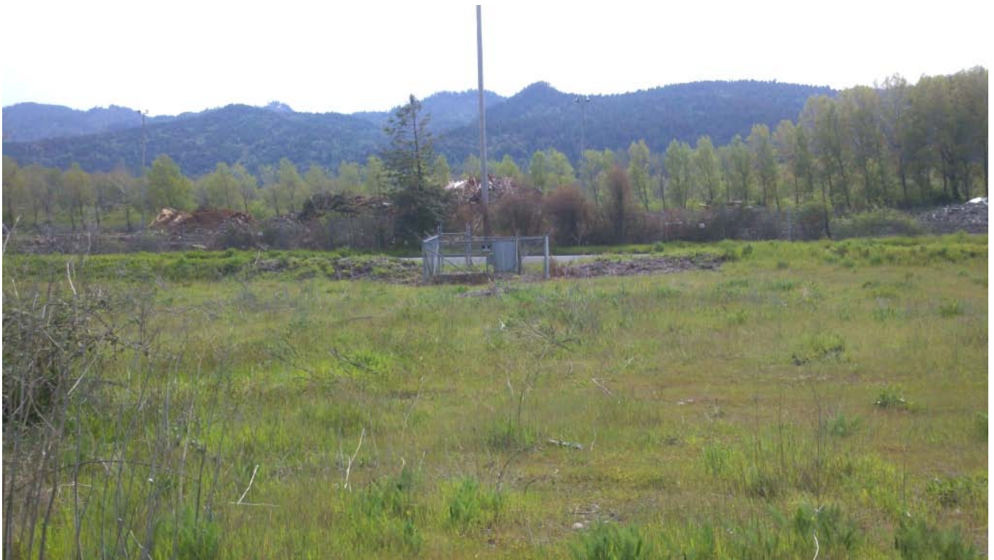
Photograph No. 6: Photo taken looking south at the City's Parcels (APN 312-161-015 and -018), and the pump station between the two, near Taylor Way.
