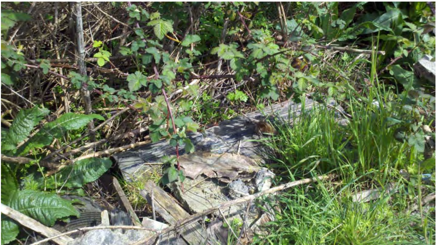
Photograph No. 36: Photo taken of fill material on City parcel APN 025-201-002.
