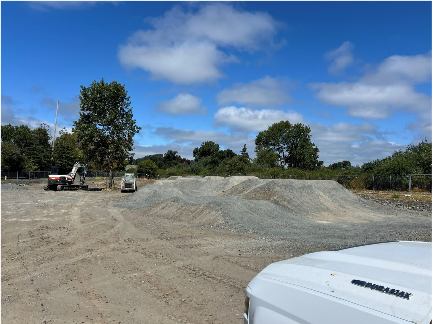
Installing base rock on compacted earthwork
